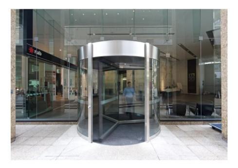
As part of the extensive ground floor building refurbishment to the plaza entry of NAB House, record Automatic Doors was engaged to provide a new revolving door entry. This required alteration works to the existing frameless glazing and a new automatic swing door entry, featuring the DFA 127 automatic swing door operator mounted under the slab to allow for a full frameless glass appearance.
